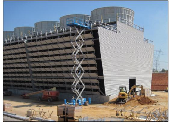
The new cooling tower at the Browns Ferry Nuclear Power Plant is the largest in the world made of composite materials.
